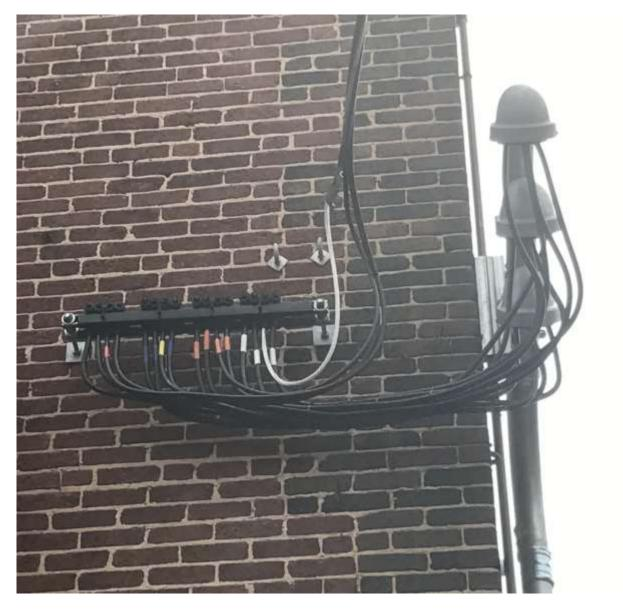
For overhead services containing multiple conductors per phase, EPB will supply a mounting bracket for the PED connectors as seen above. The customer is responsible for mounting the bracket, leaving sufficient length at the weather head, and correctly marking the load side phasing.
