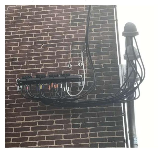
For overhead services containing multiple conductors per phase, EPB will supply a mounting bracket for the PED connectors as seen above. The customer is responsible for mounting the bracket, leaving sufficient length at the weather head, and correctly marking the load side phasing.
